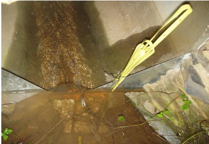
Figure 13: Weir at Culvert
