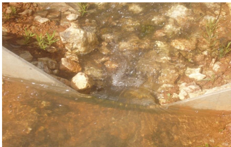
Figure 12: Weir in the overflow of the Valleygarden Lake
