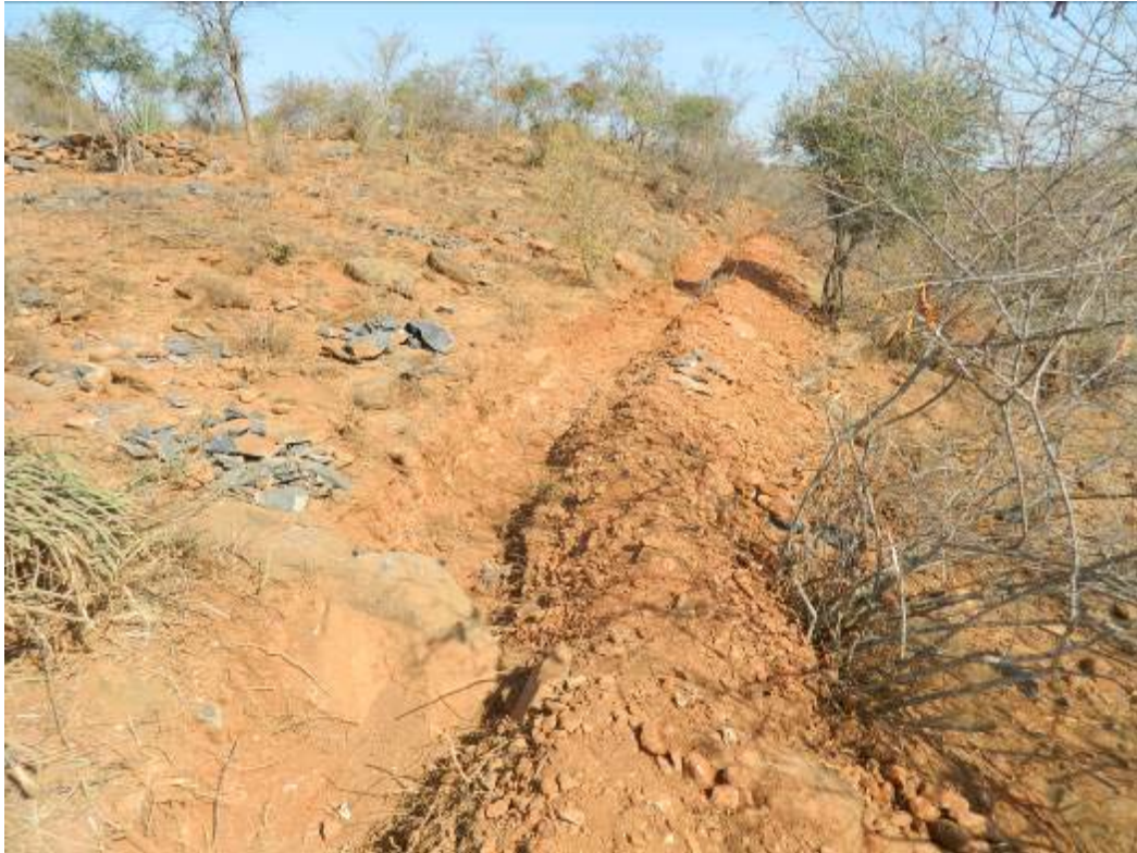
First swale on plateau ridge avoids runoff downhill
