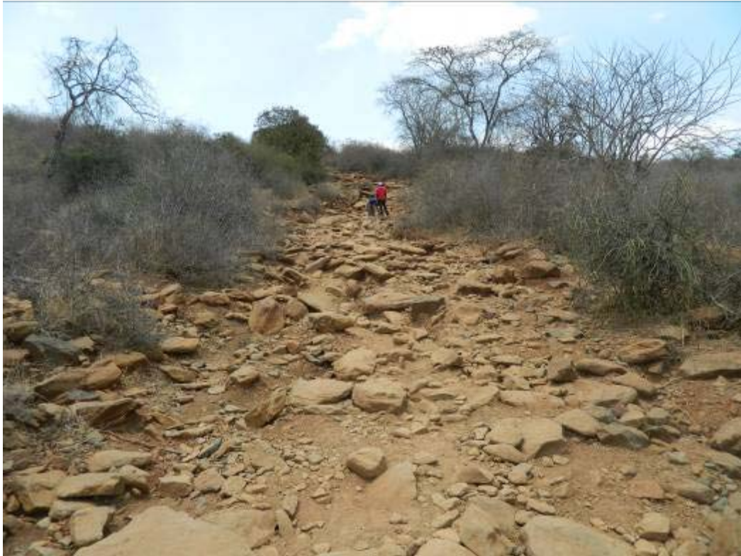
Heavy erosion on steeper part of same road
